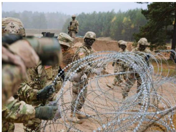
Paratroopers emplace the third strand of concertina wire on a Triple Standard Concertina wire (TSC) obstacle. Photo by LTC John Hall, November 2017.
