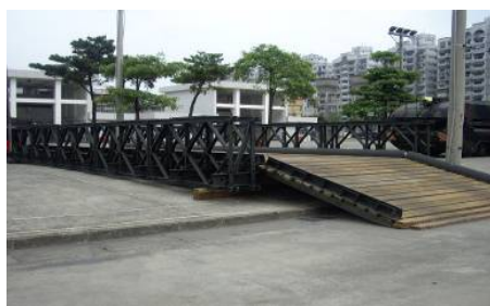
(a) M2 桁橋
