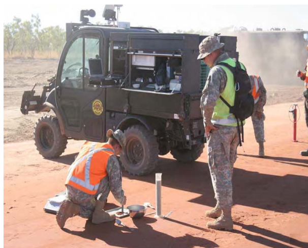
圖 17：為進行鋼珠密度試驗與 Clegg 衝擊試驗實景 參考資料：Travis A. Mann, JOINT RAPID AIRFIELD CONSTRUCTION TECHNOLOGY DEMONSTRATION, Engineer Research and Development Center, USACE,2009,p93.
